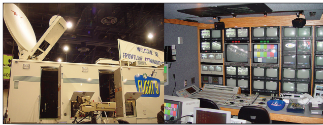
Figure 3.36 An actual truck similar to the model to the left. This truck has three 350W Ku uplink transmitters.
